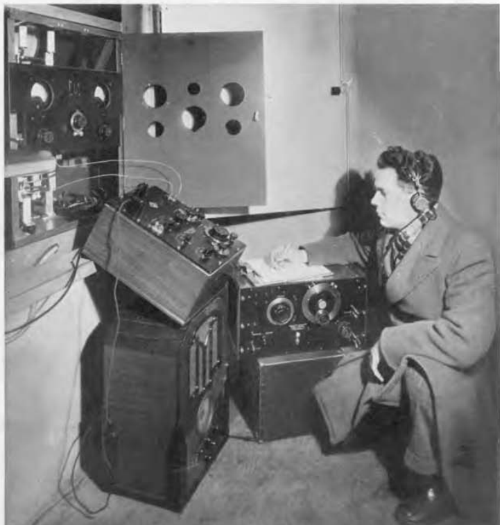
FIGURE 6. This photograph shows the radio-frequency bridge, the modulated oscillator, and radio receiver set up in the "dog house" at the base of the antenna. The equipment at the extreme left of the picture includes the impedance-matching networks and meters for reading antenna current
